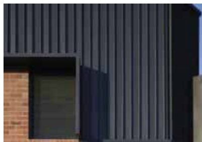
COLORBOND "LYSAGHT LONGLINE" CLADDING. COLOUR TO BE SPECIFIED.
